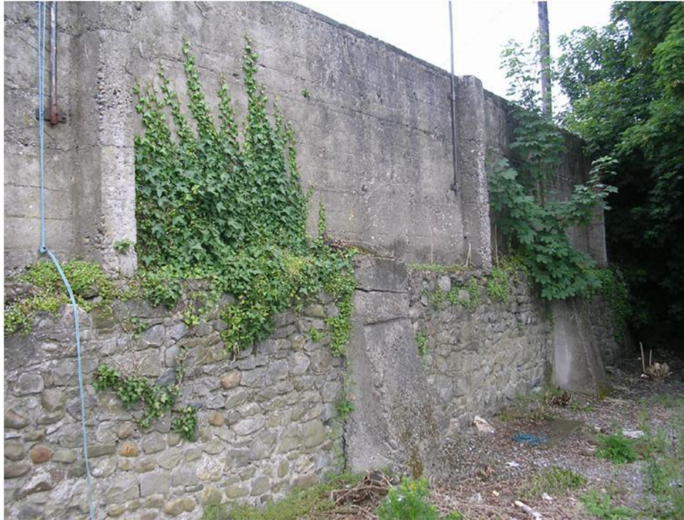
Plate 2: Northern face of wall at AH 2
