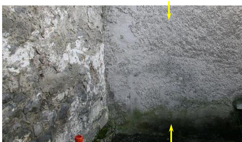
Plate 187: South-eastern corner of building with change in face indicated
