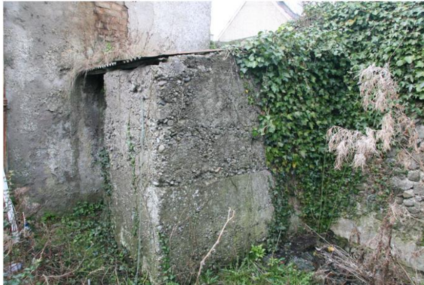
Plate 77: Concrete structure at rear of 20 Vicar Street
