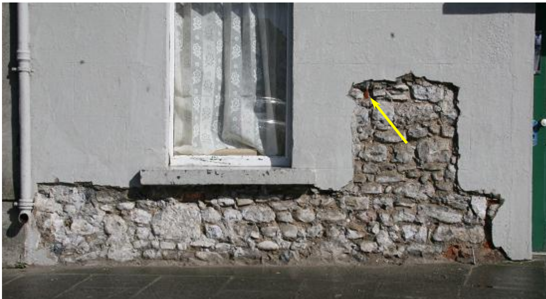
Plate 182: Opening in front facade of number 22 Vicar Street
