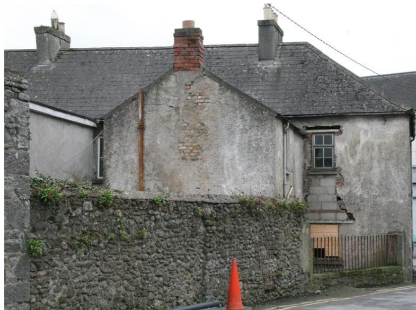
Plate 15: Rear elevation of 20 Vicar Street
