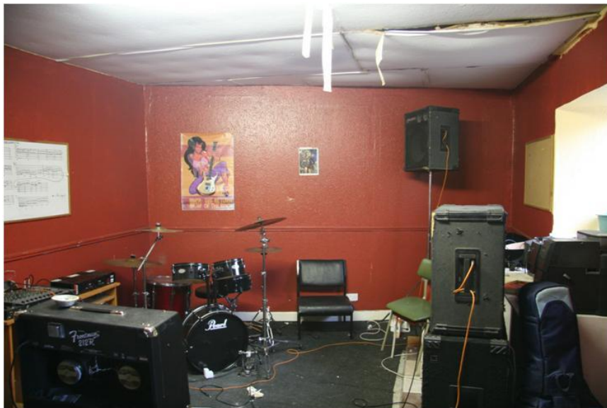
Plate 162: View southwards along larger room
