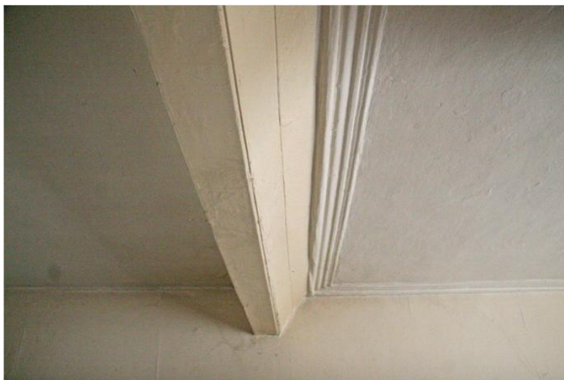
Plate 93: Timber beam in large room, with cornice at right
