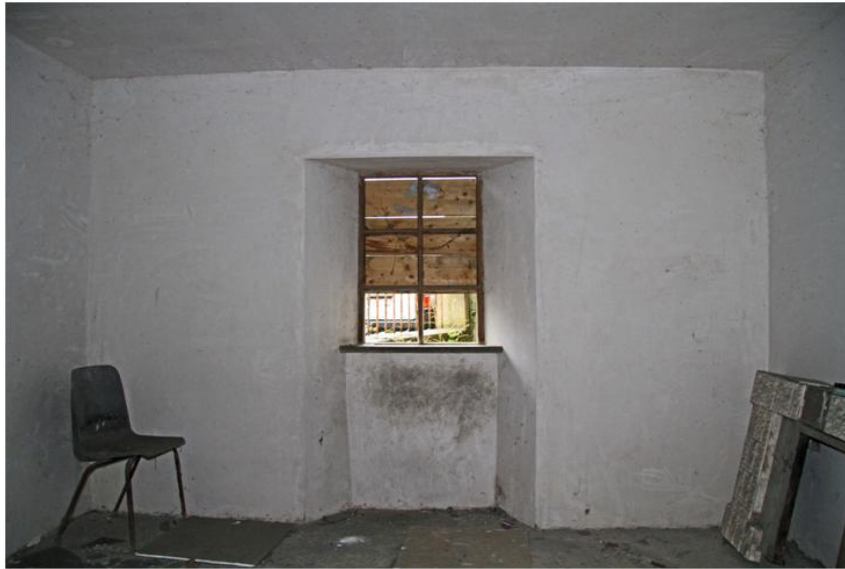
Plate 26: Rear window of large room
