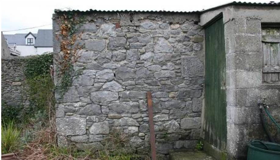
Plate 67: Southern wall of outbuilding
