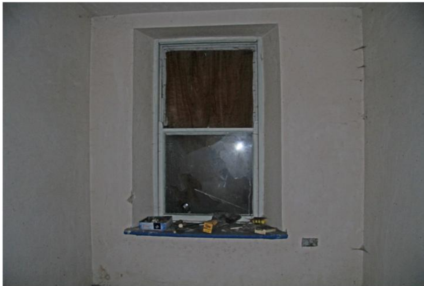
Plate 29: Front wall of small room, with window
