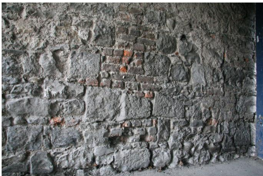
Plate 84: Detail of wall, with brick at back of hearth
