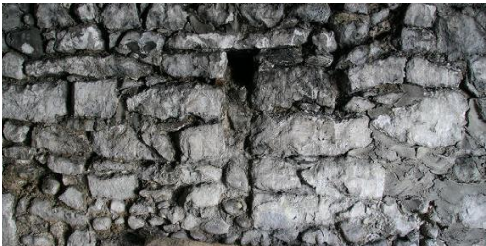
Plate 173: Ventilation slit seen within the shed
