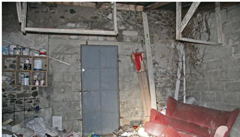
Plate 75: Interior of doorway on northern wall of outbuilding
