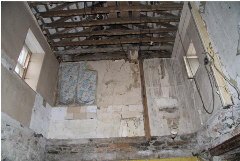
Plate 49: Return at upper floor level, looking to rear
