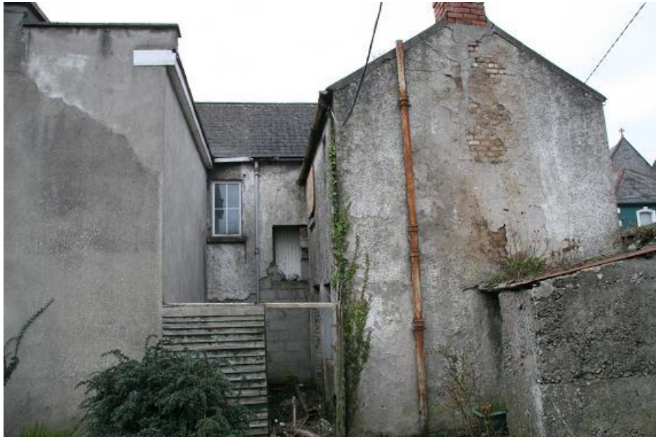
Plate 63: Rear view of 20 Vicar Street, with return of number 21 on left
