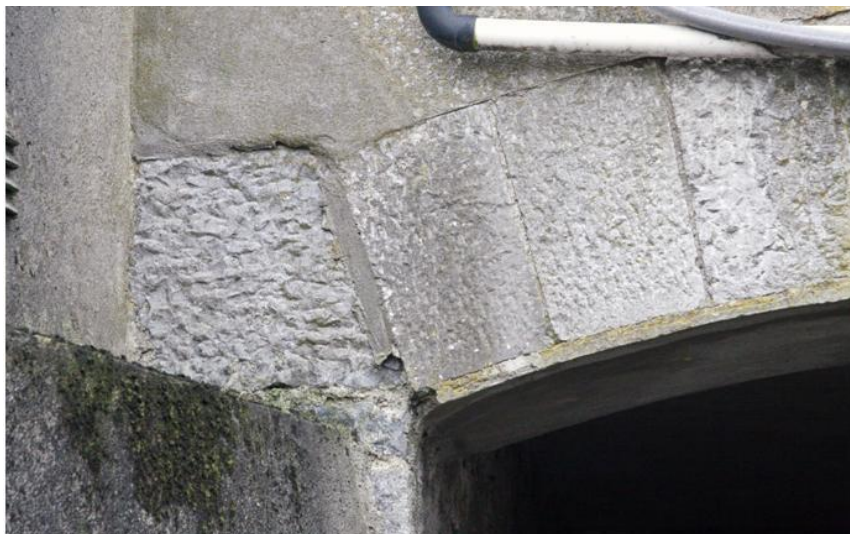
Plate 82: Detail of skewback on arch
