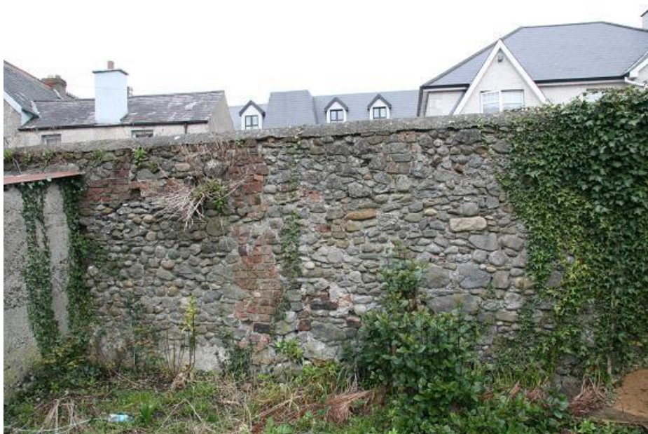
Plate 64: Part of northern boundary wall, close to house
