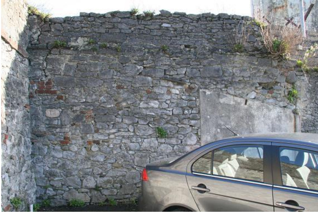
Plate 174: Central section of southern boundary, seen from car park
