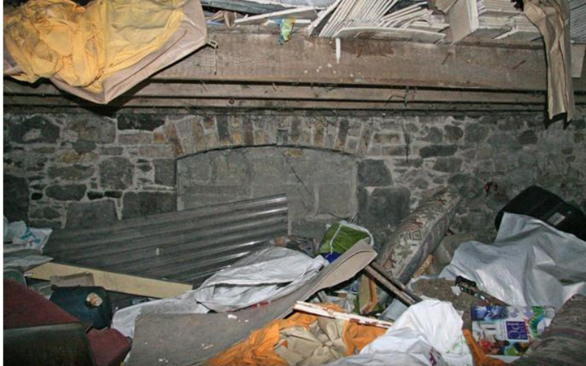
Plate 74: Interior of arch on southern wall of outbuilding
