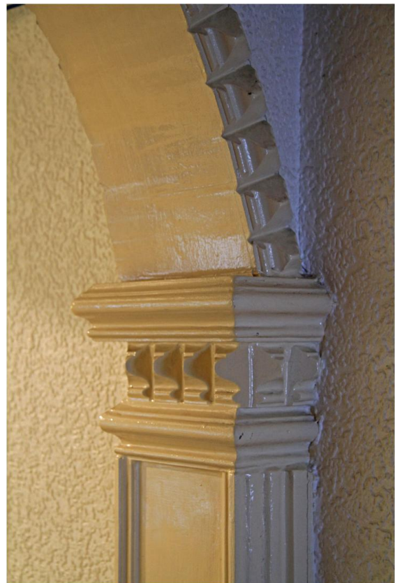
Plate 131: Detail of spring of arch and capital of pilaster
