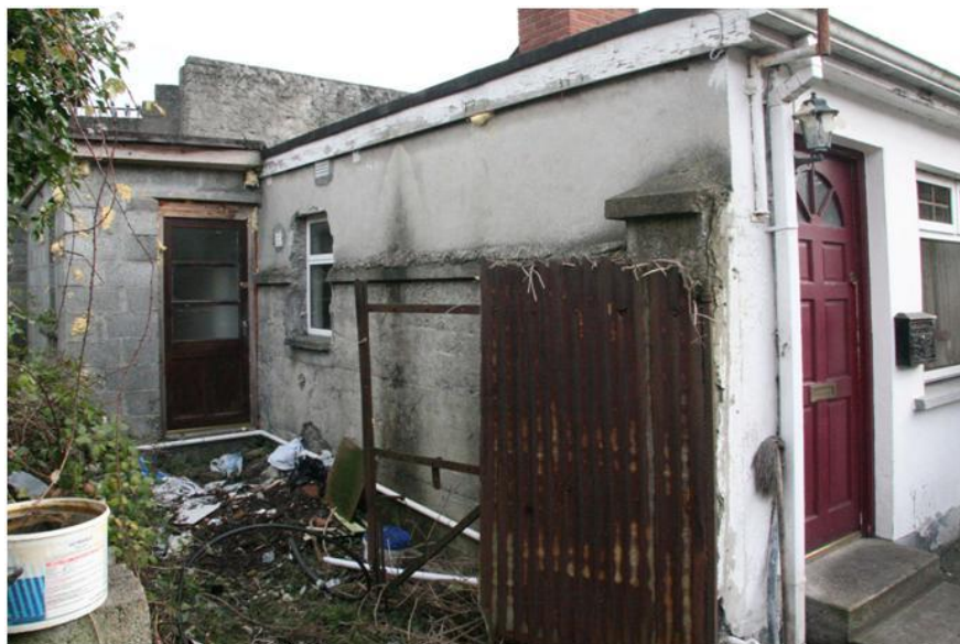
Plate 125: Northern side of flat-roofed building.
