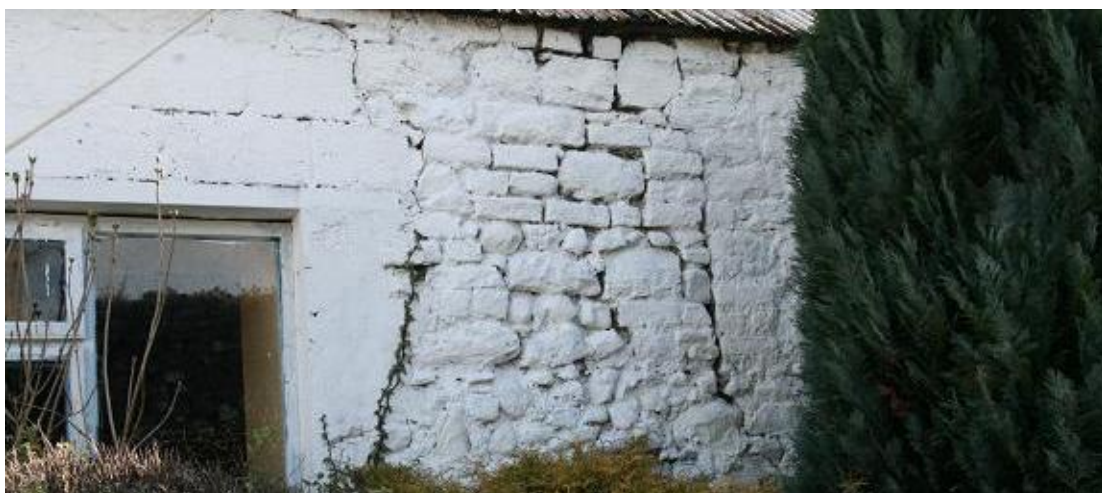
Plate 160: Area to right of window of shed A
