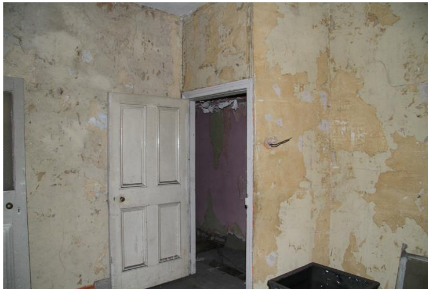
Plate 39: Doorway to front room 1 at first floor level
