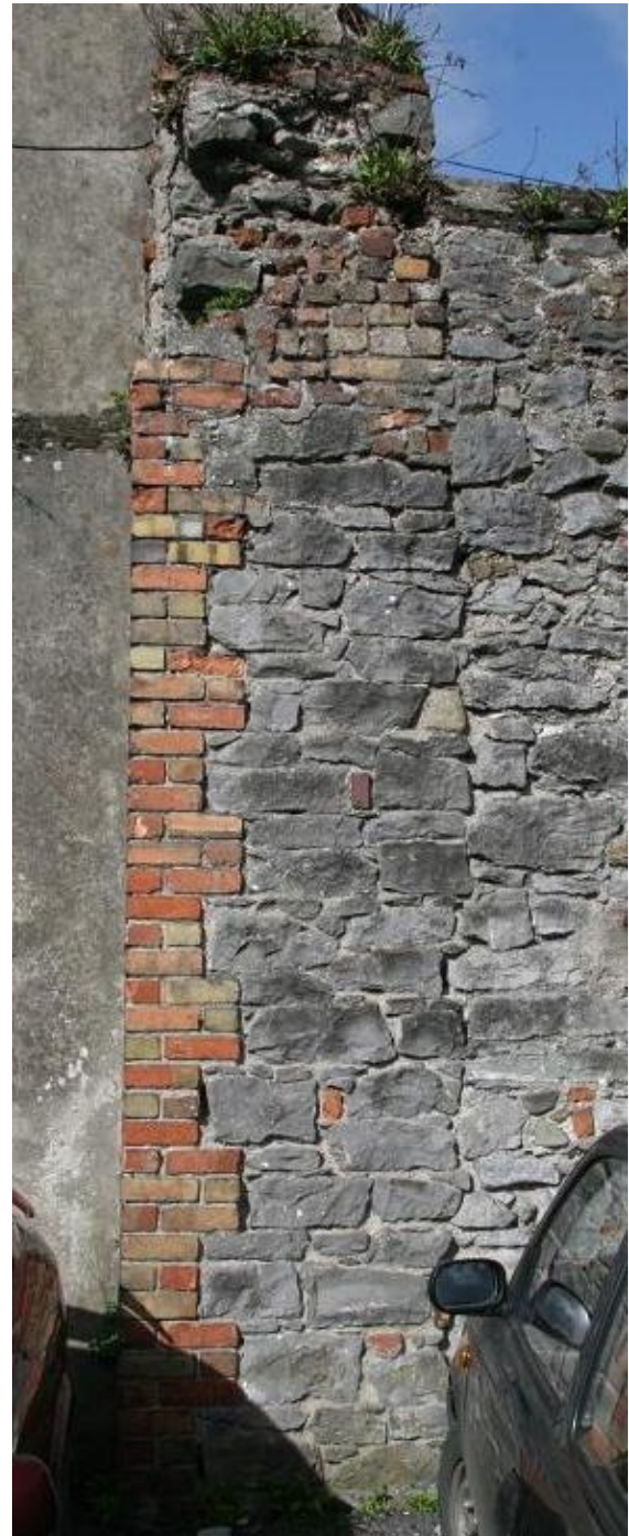
Plate 179: Western end of southern boundary wall
