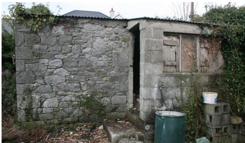
Plate 72: Eastern side of outbuilding, with concrete porch
