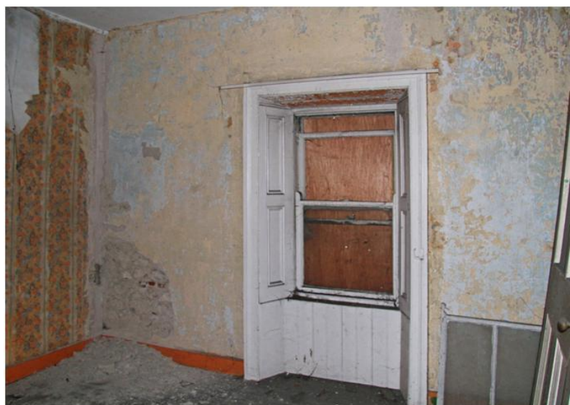
Plate 40 (above): Front wall of room
