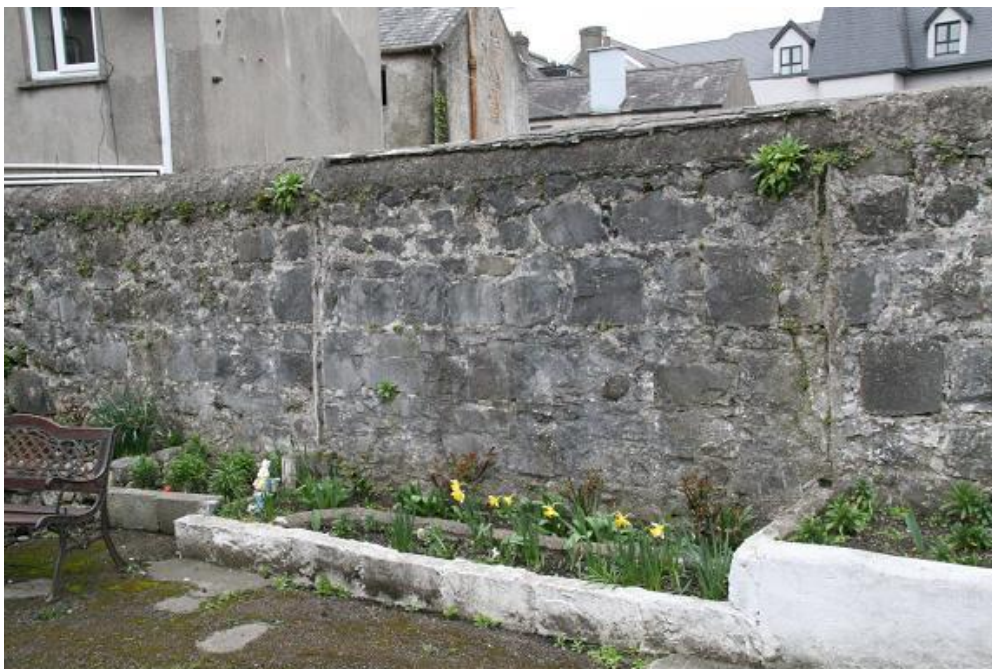
Plate 170: Northern boundary wall
