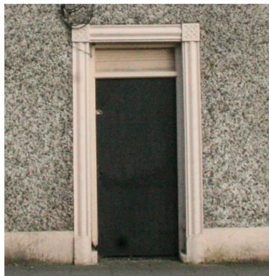
Plate 13: Front doorway to number 20
