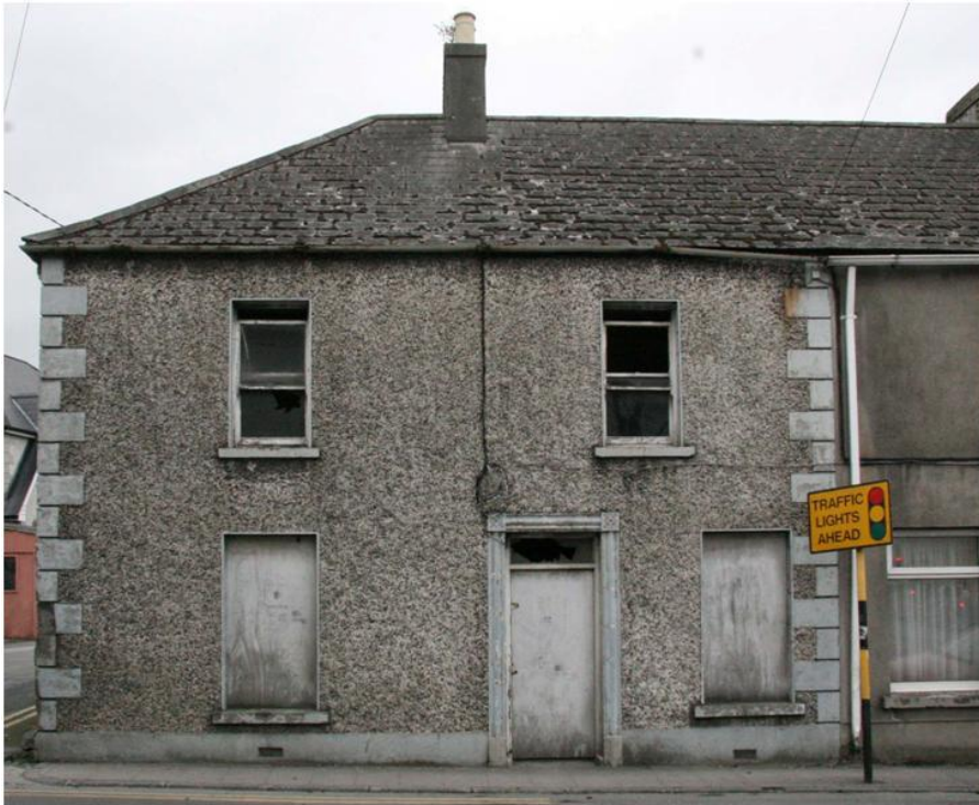
Plate 12: Front facade of 20 Vicar Street
