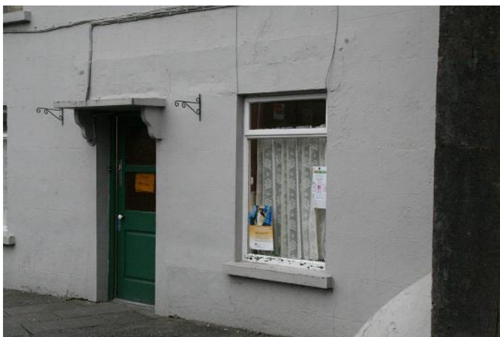
Plate 181: Southern part of ground floor facade showing shopfront
