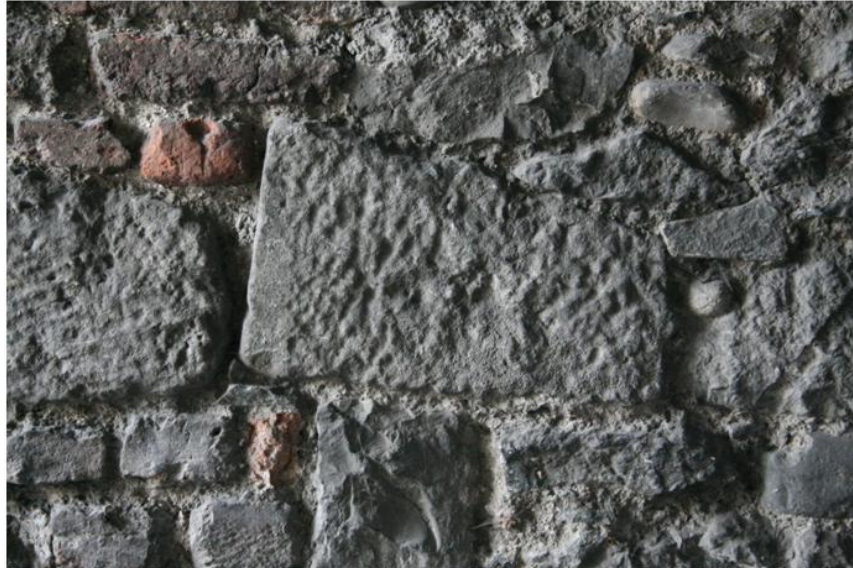
Plate 85: Detail of reused dressed stone in wall at arch
