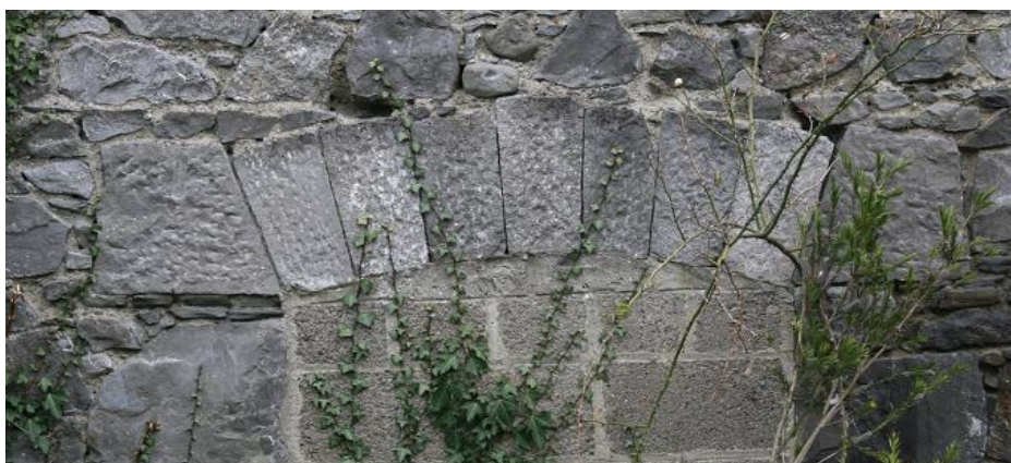
Plate 71: Detail of arch of doorway
