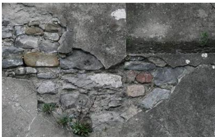
Plate 184: Masonry at chimney stack
