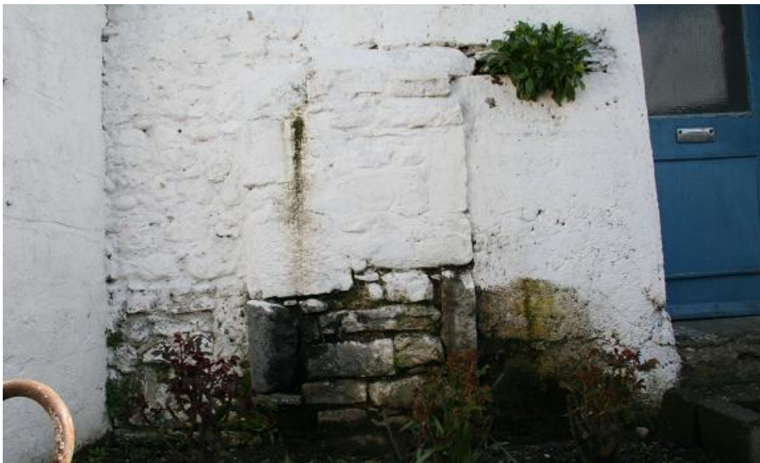
Plate 158: Buttress at front of shed A
