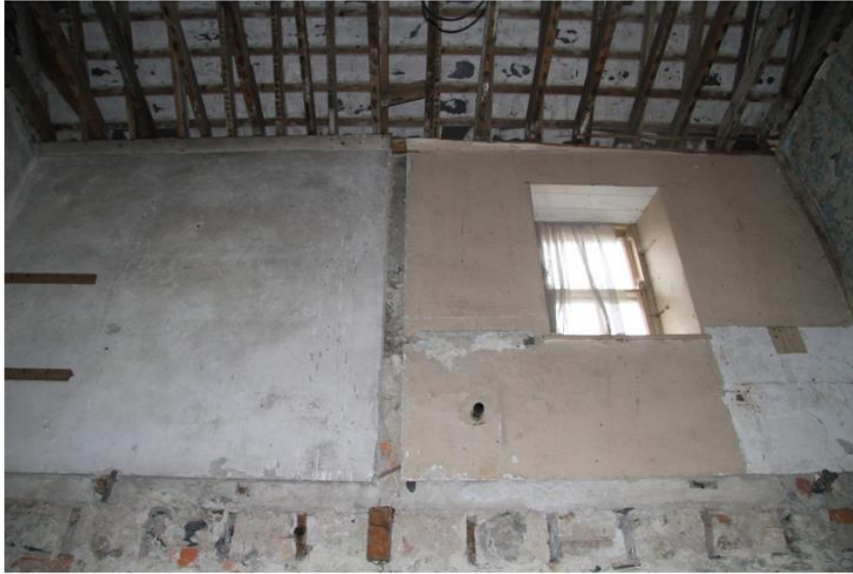
Plate 52: Western wall of return at first floor level
