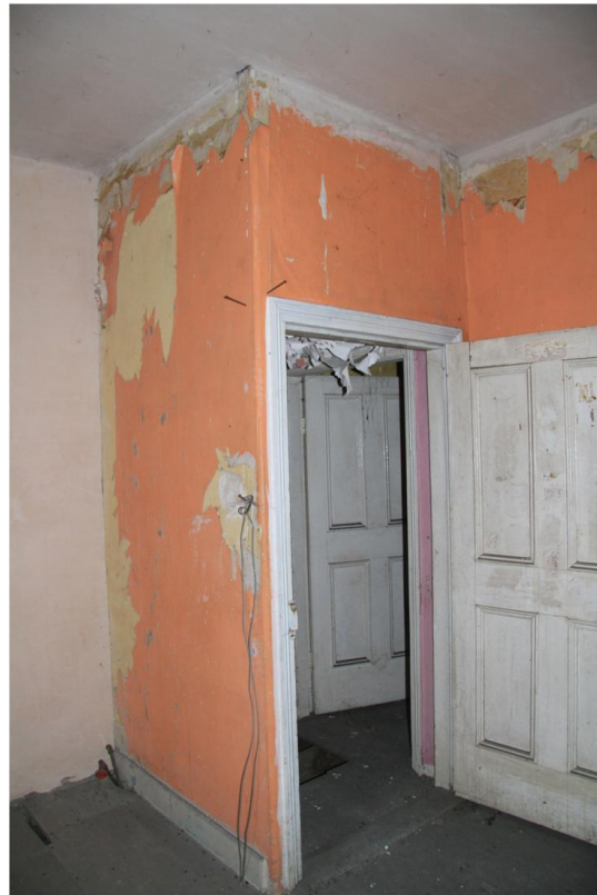
Plate 46: Door to rear room
