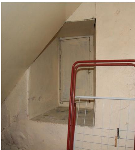
Plate 140: Window ope beneath stairs
