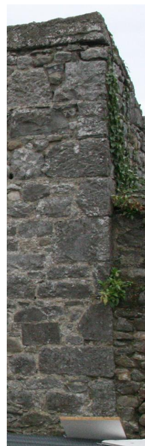
Plate 66: North-western corner of shed
