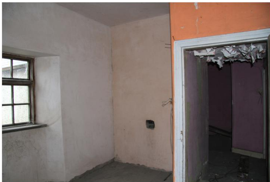
Plate 47: Window and blocked hearth in rear room
