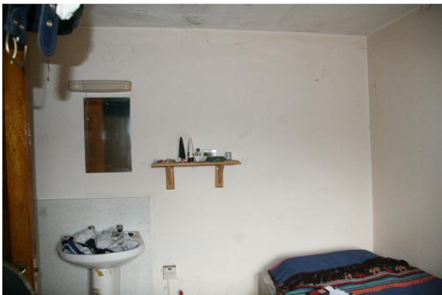
Plate 110: View to north in room in return
