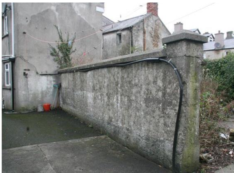
Plate 122: Northern boundary wall
