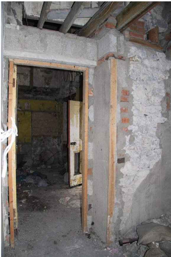
Plate 23: Doorway to return at rear
