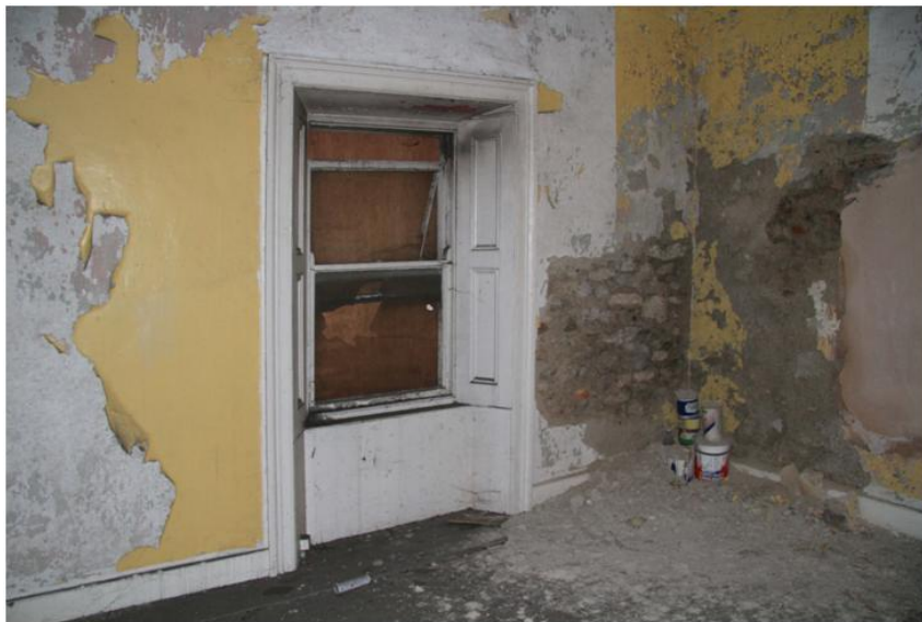
Plate 42: Window in front room 2
