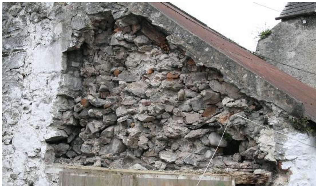
Plate 168: Collapsed gable at eastern end of shed D
