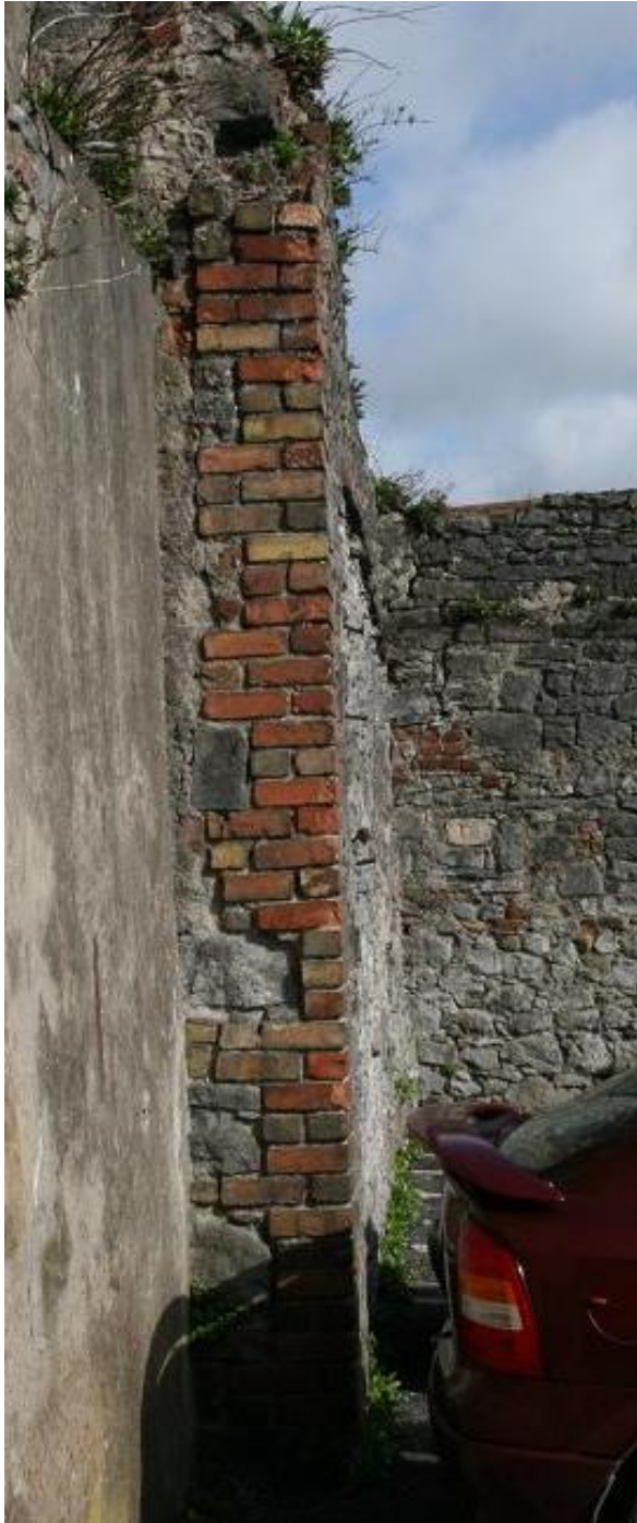
Plate 178: Western end of southern boundary wall, at rear corner of house
