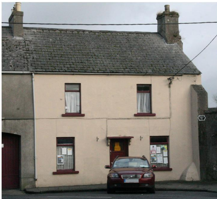
Plate 126: Front facade of 22 Vicar Street
