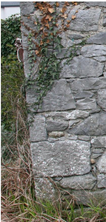
Plate 68 (left): Details of hammer-dressed stone quoins at corner
