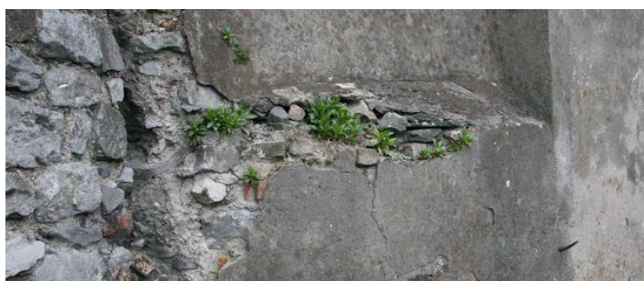
Plate 185: Masonry at base of gable wall
