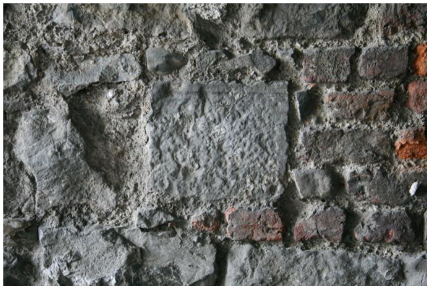
Plate 86: Detail of reused dressed stone in wall at arch
