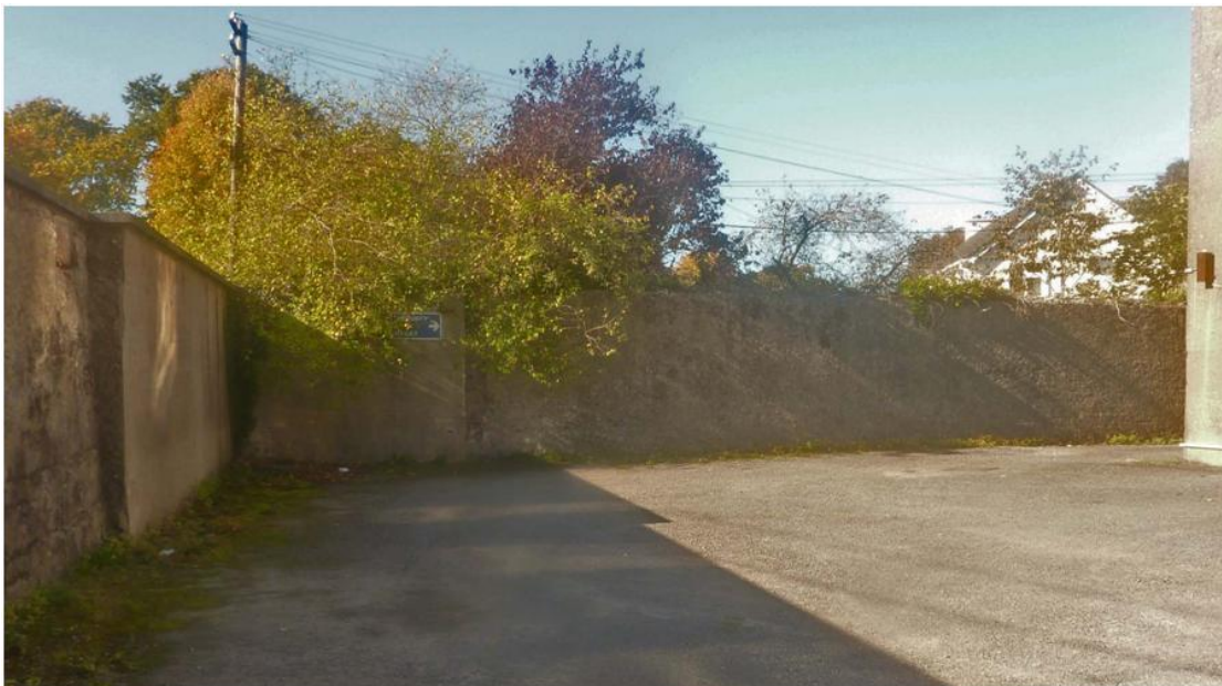
Plate 7: Northern end of front wall, and northern boundary wall
