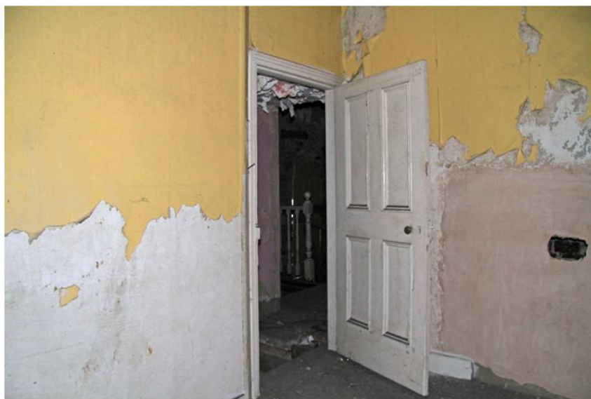
Plate 43: Door in front room 2
