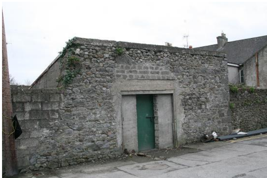
Plate 65: Shed at rear, northern face, to Mill Lane
