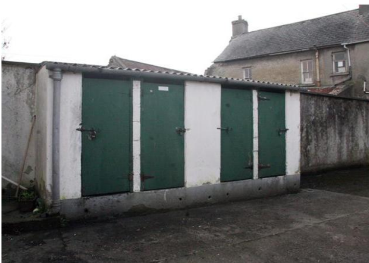
Plate 123: Storage sheds at rear of 21 Vicar Street
