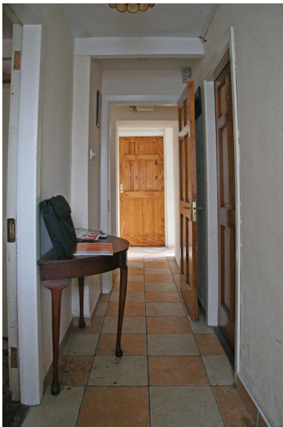
Plate 88 (left): View to rear of corridor
