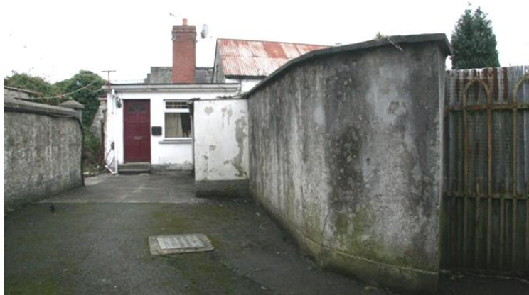
Plate 121: Southern boundary wall, at right
