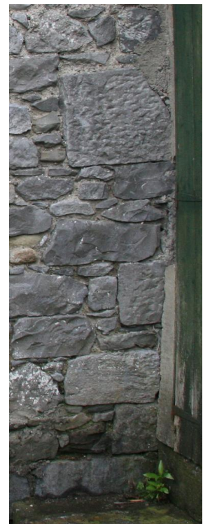
Plate 69 (right): Details of hammer-dressed stone at former opening
