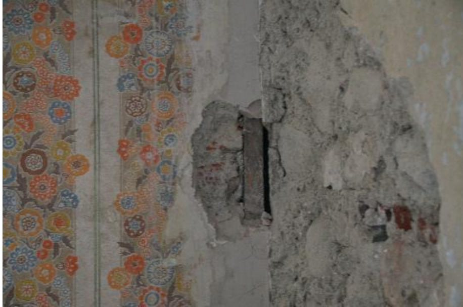
Plate 58: Party wall between numbers 20 and 21 at first floor level
