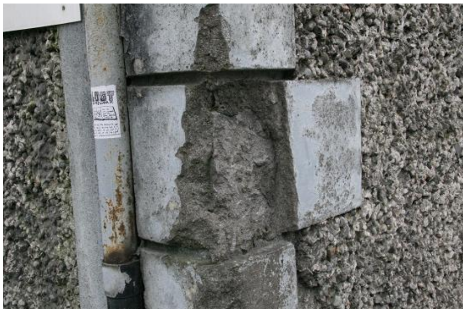
Plate 62: Front corner of 20 Vicar Street, at north-western corner
