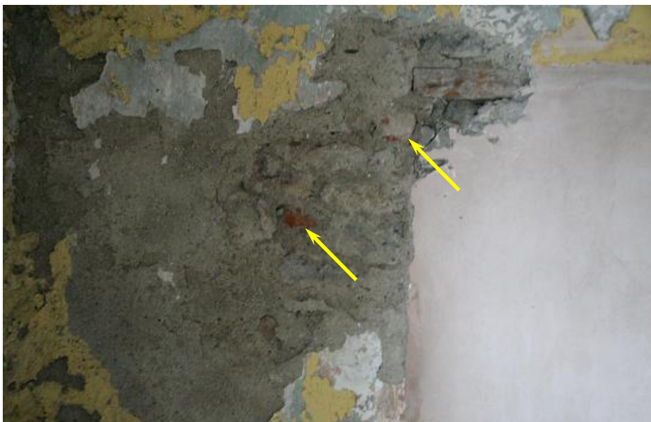
Plate 57: Inner face of northern end wall of number 20 Vicar Street The timber lintel is seen to the right of the upper arrow, at a higher level
