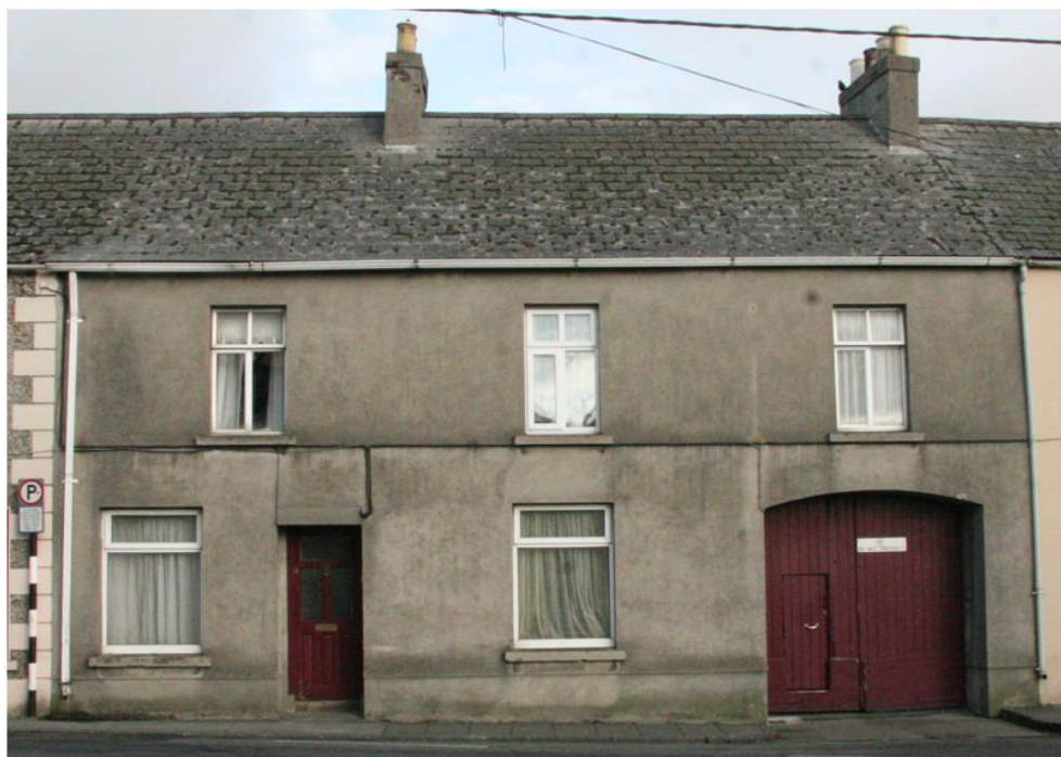
Plate 78: Front facade of 21 Vicar Street
