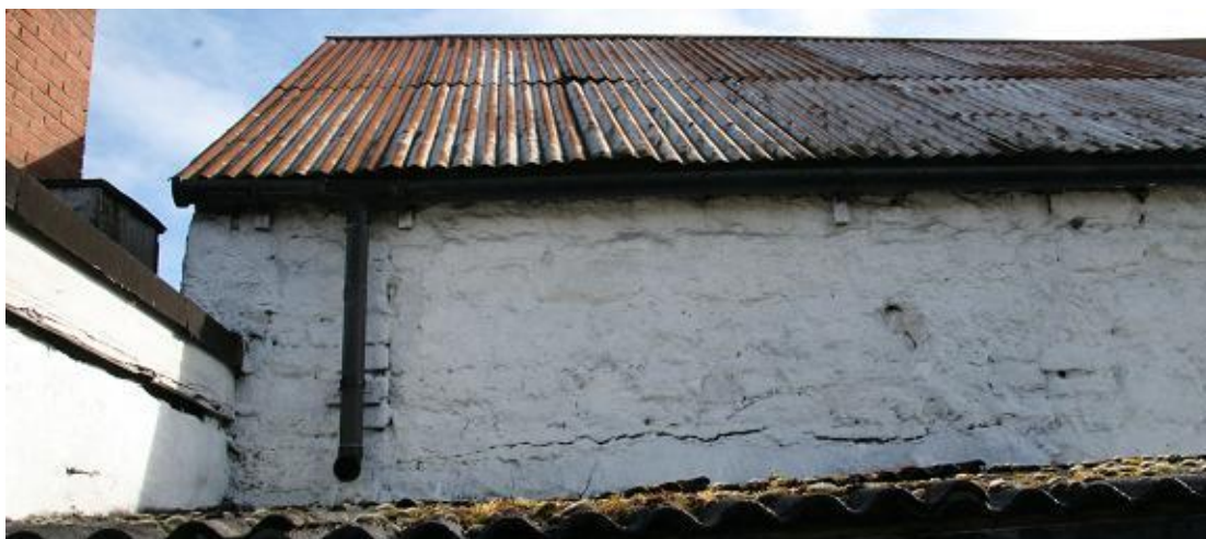
Plate 156: Northern end of building, above shed B
