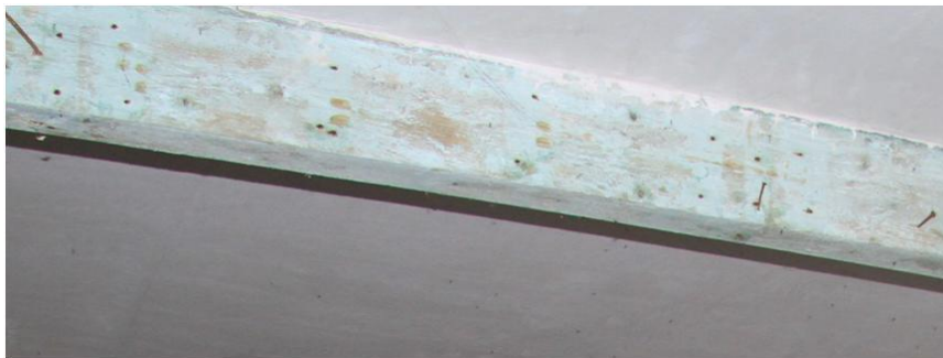
Plate 27: Detail of timber beam crossing ceiling
