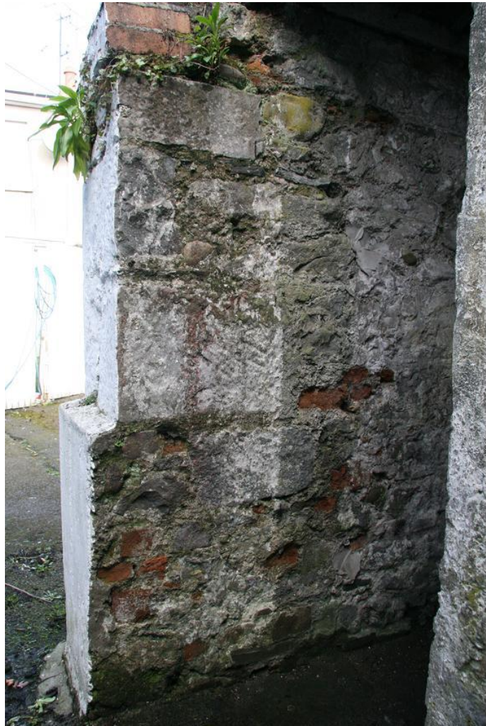
Plate 169: Pier at end of shed D with dressed stone in mid section
