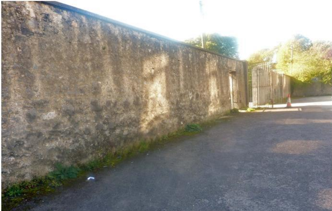
Plate 6: Internal face of wall at road frontage
