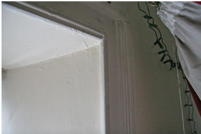
Plate 102: Surviving architrave and window lining
