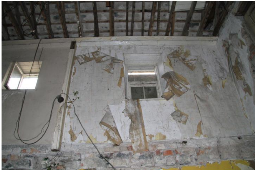
Plate 51: East-facing side wall of return
