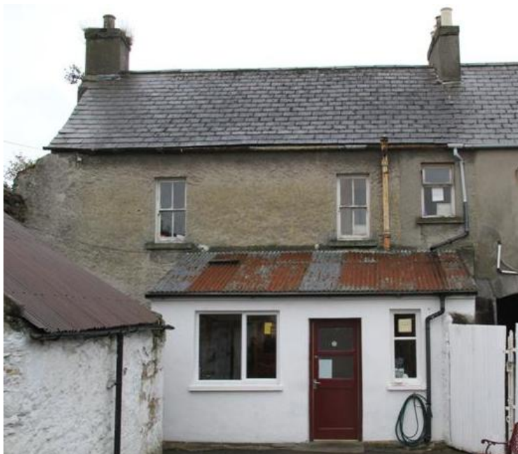
Plate 129: Rear facade of 22 Vicar Street
