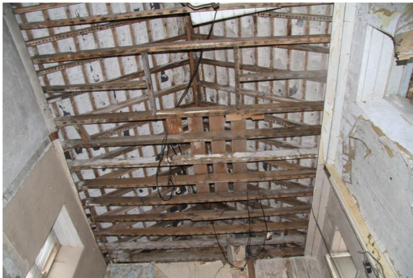
Plate 53: Roof structure in return
