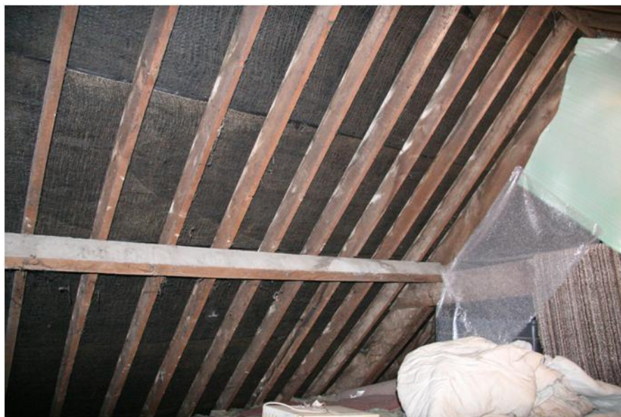
Plate 114: Underside of roof in attic of 21 Vicar Street
