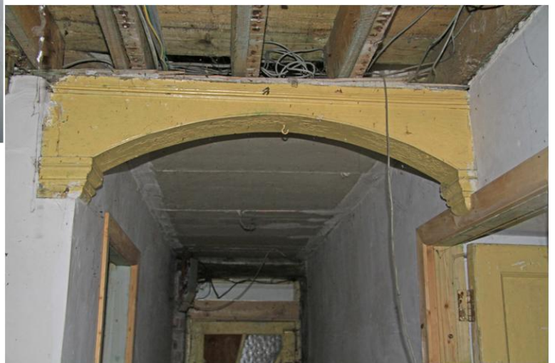
Plate 21: Timber beam over hallway
