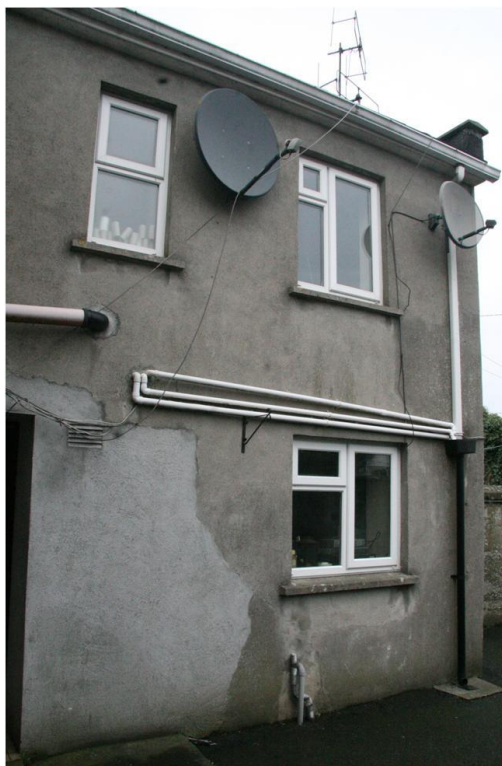
Plate 80: Southern side of return
