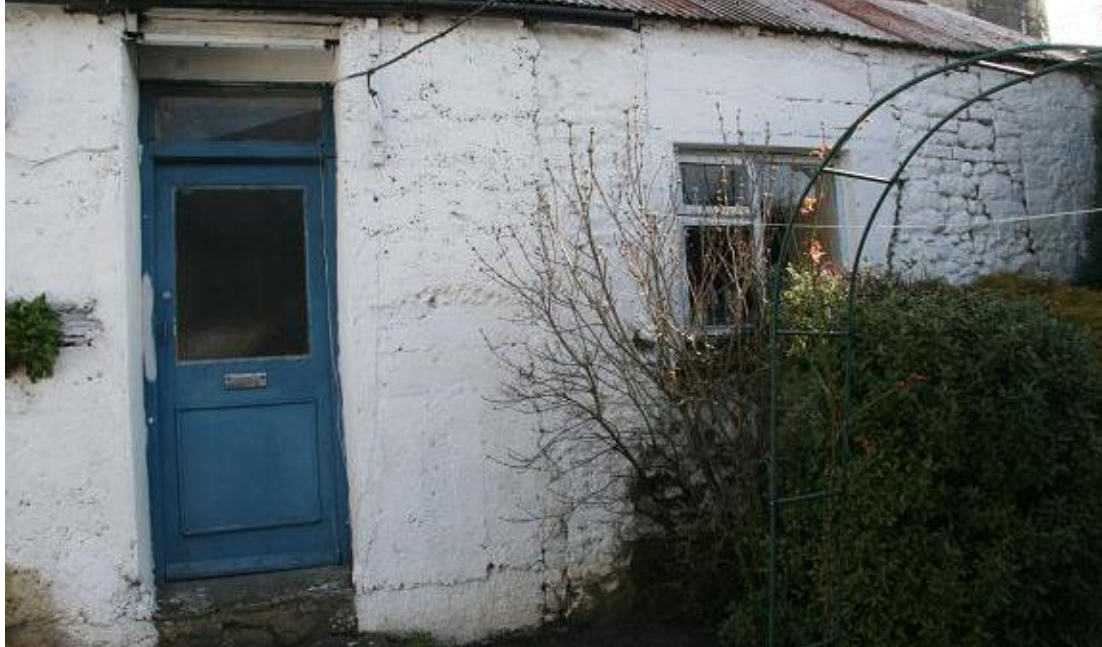
Plate 159: Area to right of door of Shed A
