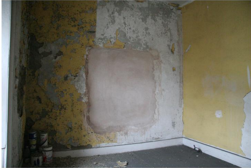
Plate 44: Blocked up in external wall of front room 2
