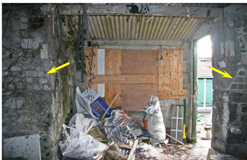
Plate 76: Ope on eastern wall, with skewbacks marked with arrows
